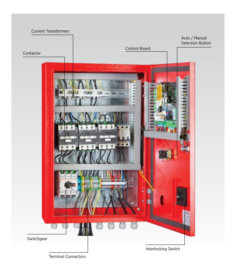
Figure 2. EN 12845 Electric Control Panel- Internal View
